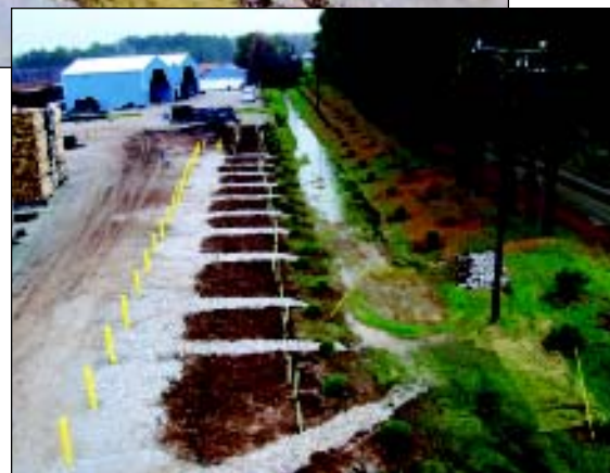
ABOVE: A wetland was constructed after remediation in a downstream portion of the on-site drainage. RIGHT: Post-remediation is evident at the on-site drainage ditch, which includes a buffer zone (mulched area), the DNAPL barrier (along yellow posts) and riparian zone revegetation (on both sides of the drainage ditch). Photos submitted
