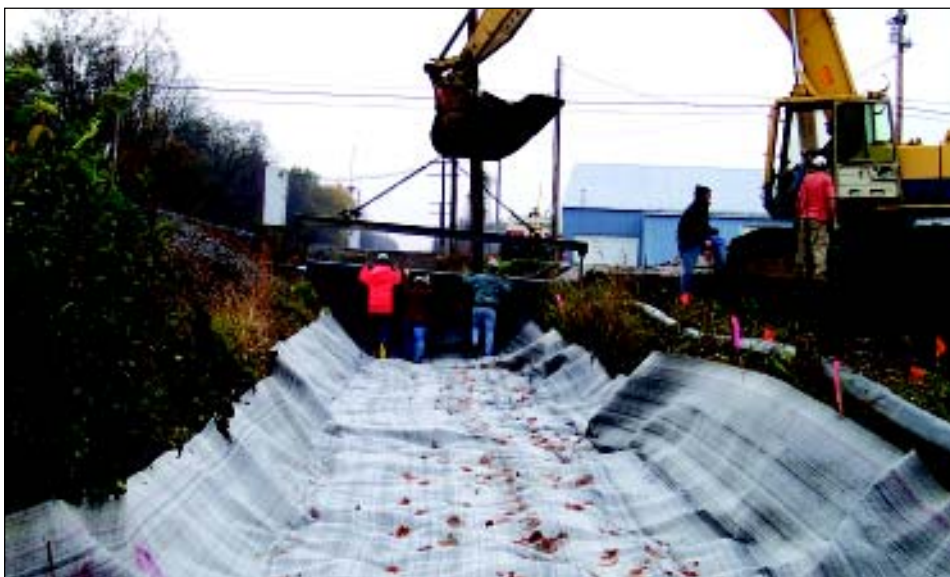
LEFT: Placement of a geosynthetic clay liner helped to isolate remaining sediments from the restored stream bottom. Photo submitted
