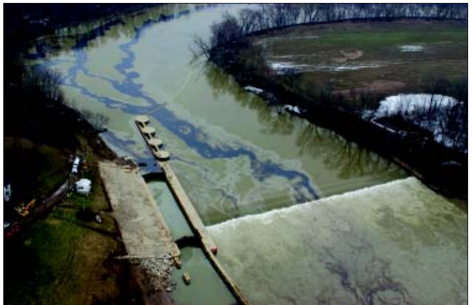
Faintly visible, a yellow boom stretches across the Kentucky River trying to hold back the oil. However, the boom was breached and oil flowed northward past the Lock and Dam 1 outside of Carrollton. Aerial photo provided by J. Hamon
