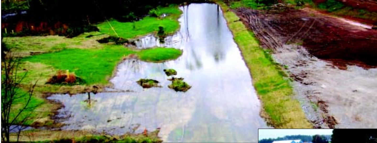
ABOVE: A wetland was constructed after remediation in a downstream portion of the on-site drainage. RIGHT: Post-remediation is evident at the on-site drainage ditch, which includes a buffer zone (mulched area), the DNAPL barrier (along yellow posts) and riparian zone revegetation (on both sides of the drainage ditch). Photos submitted
